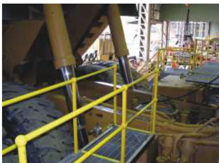
Ladder for access from the platform to the dump truck
