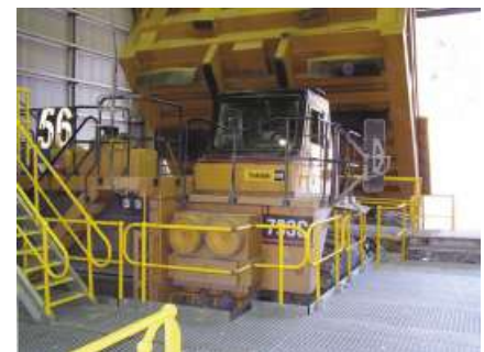
Working floor on the platform
